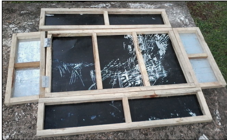
Plate 2. Portable and Foldable type Solar Dryer in Construction
